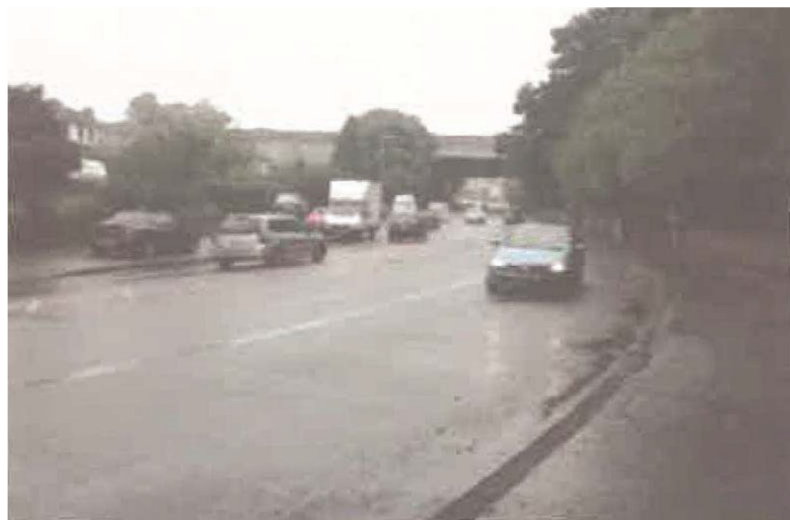
Illustration 15: M1 Motorway Bridge
